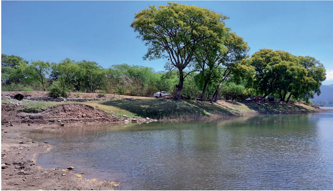
Figure 5. La Ciénaga dam 24°25'50.10''S, 65°16'41.0''W. El Carmen Department, Jujuy Province.
